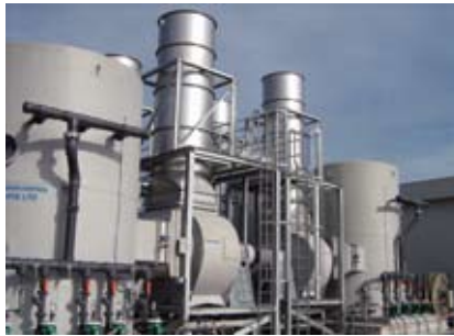
Seagate Senai Scrubber System
