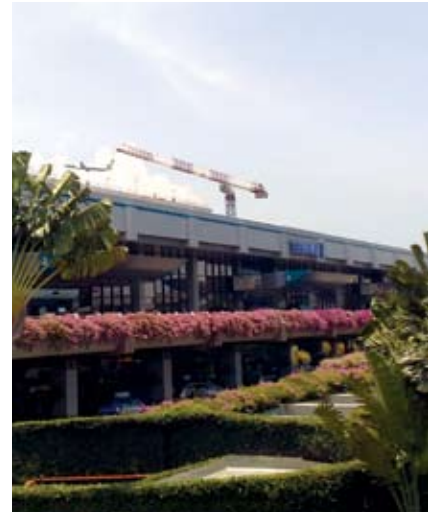
Changi Airport Terminal 1 project
