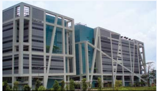
Bio-Polis ACMV Maintenance
