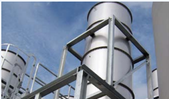
Seagate Senai Scrubber System
